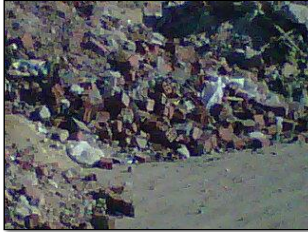
Figure 3.7: Demolition waste on site
