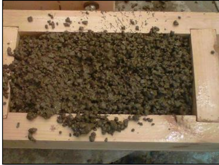
Figure 3.21: Pouring the mix into molds
